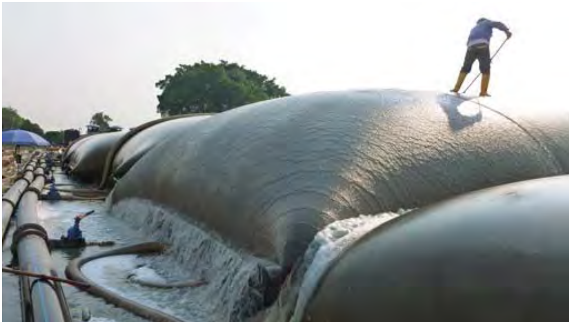
Figure 5-2 Dewatering Using Geotubes ( http://www.gowatersolve.com/geotube )
